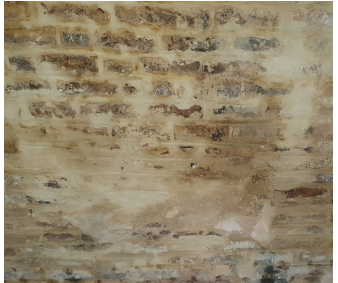
Evidence of damp in brickwork that has been pointed with Portland cement mortar
