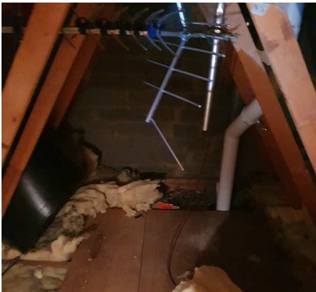
Inadequately insulated loft
