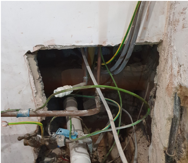
Service openings through external walls are inadequately sealed
